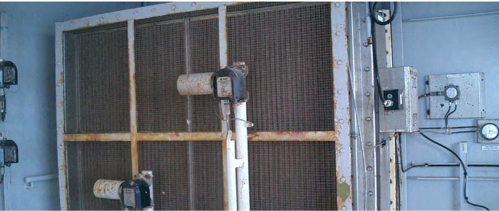
Accommodation HVAC air intake damper with gas detection
