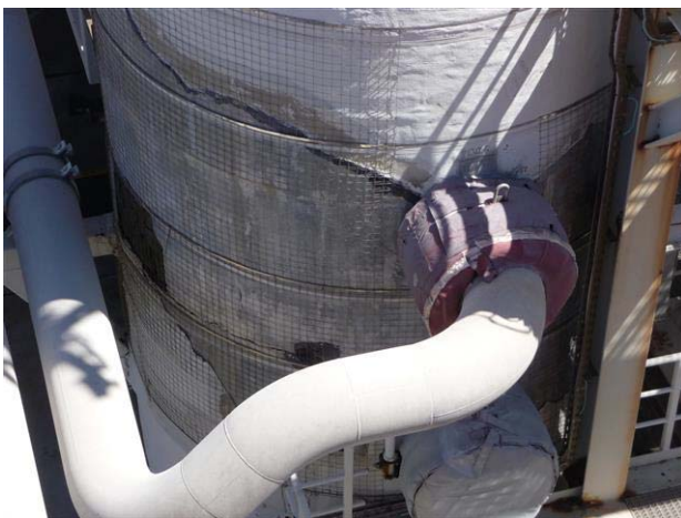
Figure 1 - Temporary Repair to PFP on the Debutaniser Column
