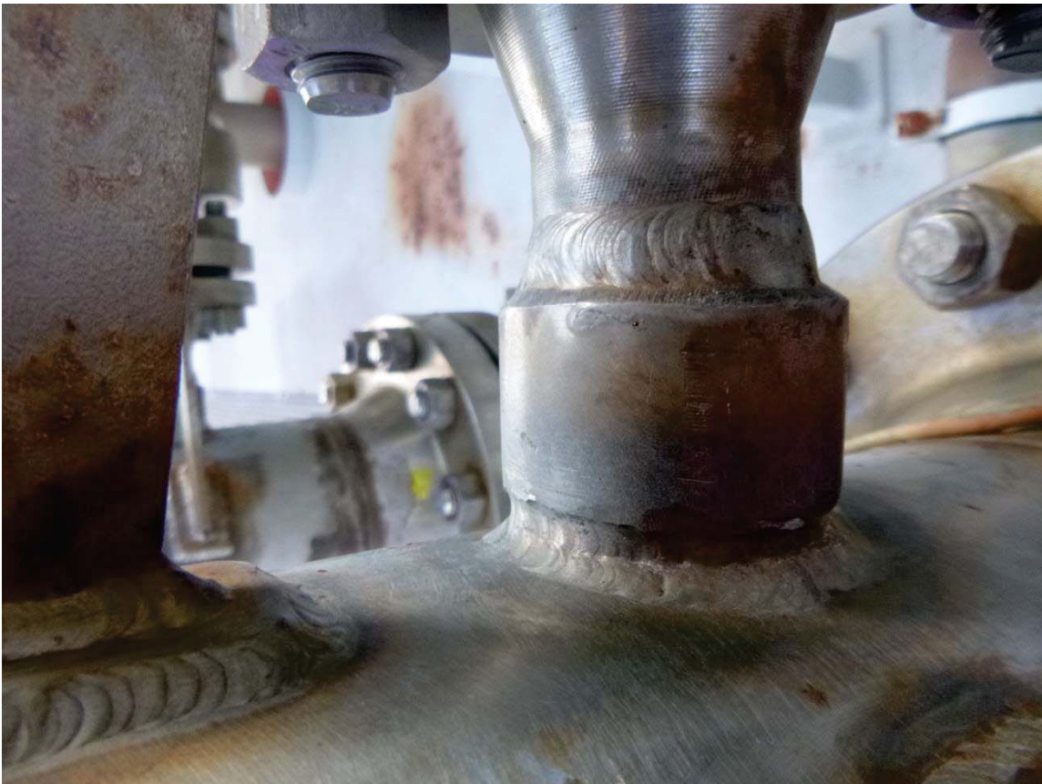
Figure 12 - 150-PG-3037-03D01-0 TP2 (Q) condition of small bore fitting weld
