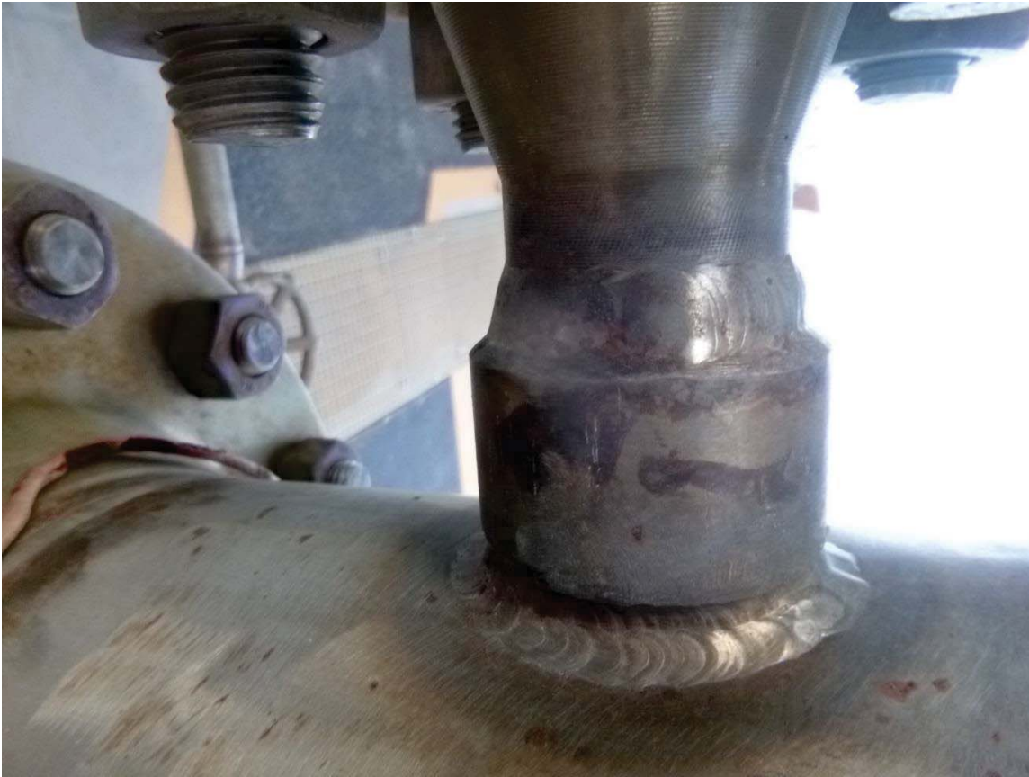
Figure 12 - 150-PG-3037-03D01-0 TP2 (Q) condition of small bore fitting weld
