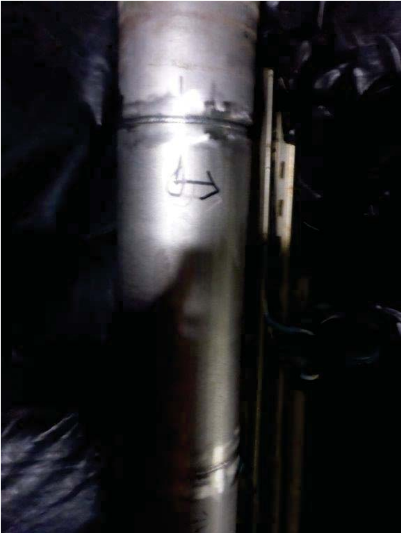
Figure 19 - Replacement spool piece on line 150-PL-3052-03D01-3 with SBF designed out
