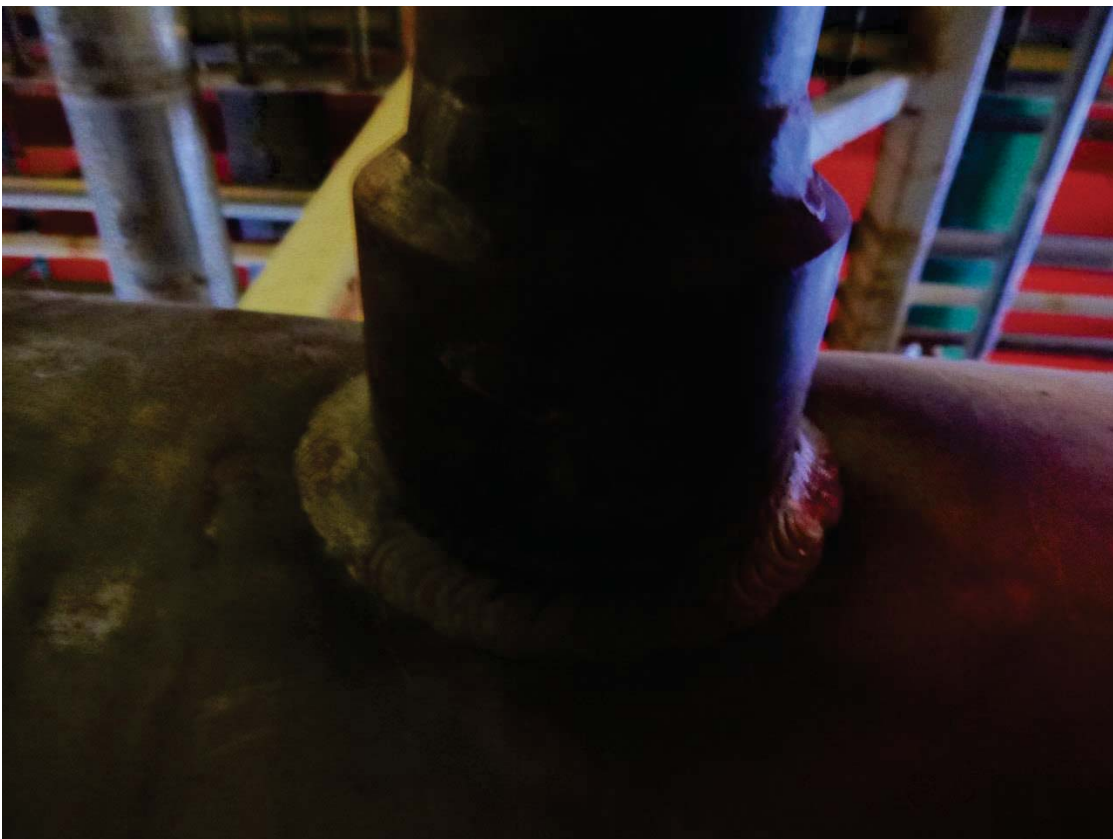
Figure 16 - 150-PL-4032-03D01-0 WOL (T) condition of small bore fitting weld
