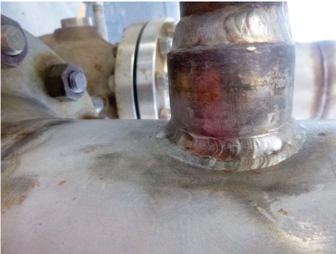
Figure 8 - 150-PG-3037-03D01-0 TP1 (P) condition of small bore fitting weld
