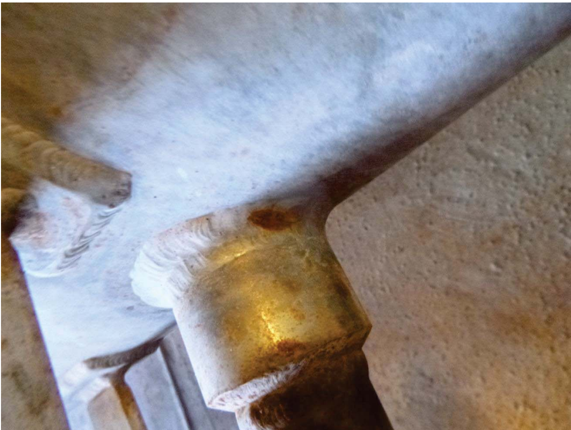
Figure 14 - 150-PL-4030-03D01-0 TP1 (H) condition of small bore fitting weld
