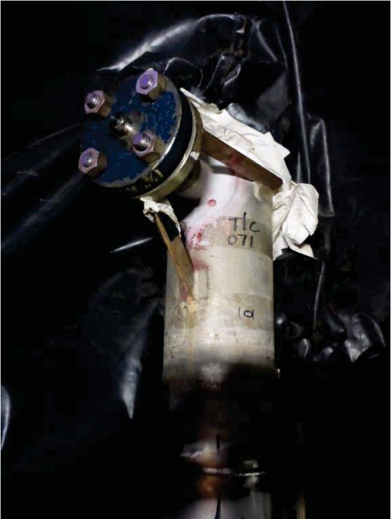
Figure 18 - Previous brace configuration at 37PI072 on line 150-PL-3052-03D01-3
