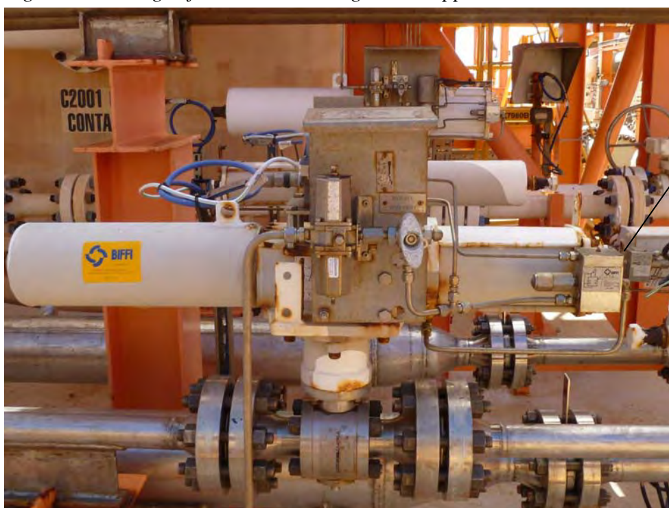
Figure 4.2 – Image of Exhaust Flow Regulator Supported on XV11420
