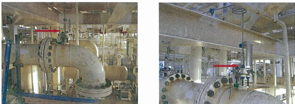
Figures 1 & 2 Pre-event Piping and Instrument Tubing arrangement at MPA 1st Stage Suction
