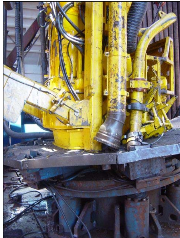
Top Drive impacted riser gimbal at rig floor level
