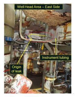
Figure 1 – Location of failed instrument line (dashed line) fitted to gas lift line between the production annulus wing valve and gas lift shutdown valve.
