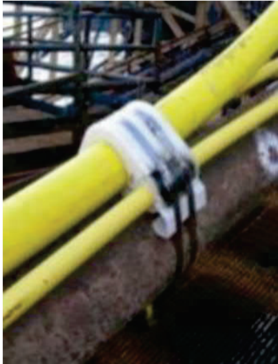
Figure 2: Piggyback clamp during construction/installation
