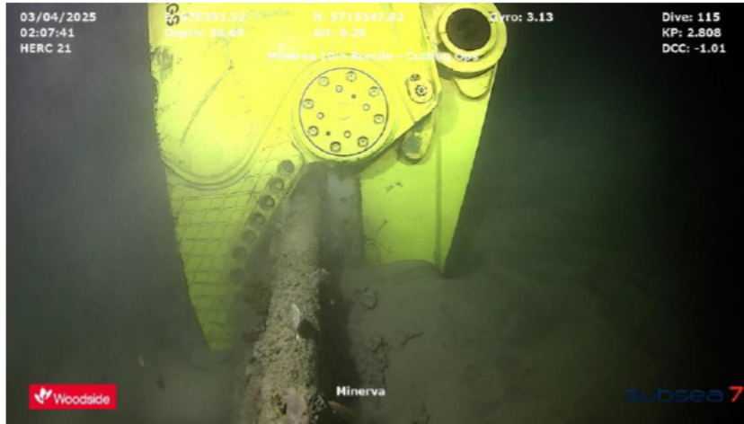
Pipeline cutting
