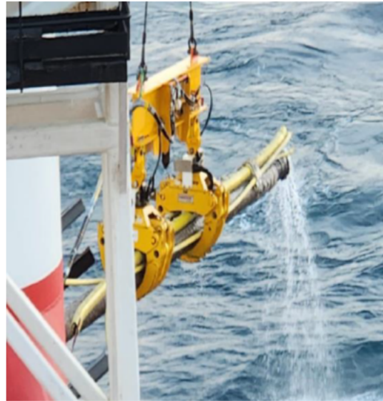
Retrieval of pipeline section
