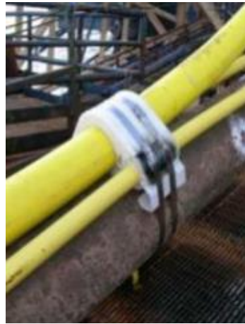
Figure 2: Piggyback clamp during construction/installation
