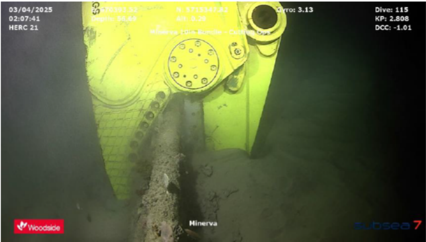
Pipeline cutting
