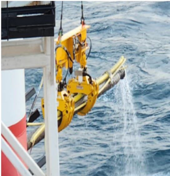
Retrieval of pipeline section
