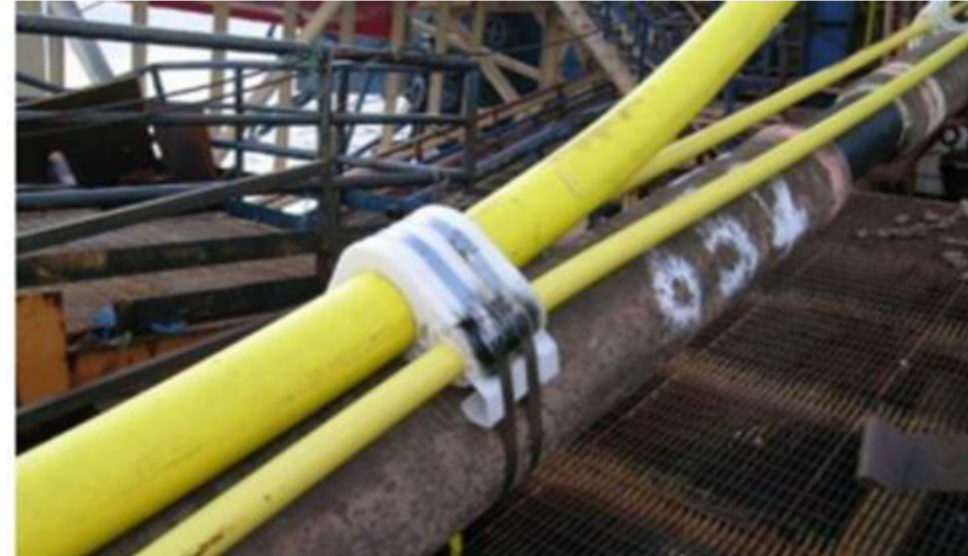
#4: An existing photo during construction showing the plastic saddle bundled together with other pipes.
