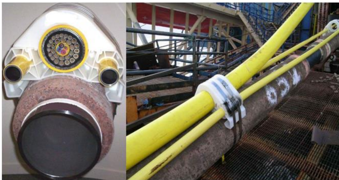
Figure 2: Photos of piggyback clamps during the installation process
