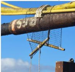
Saddle retention nets after recovery to outer
