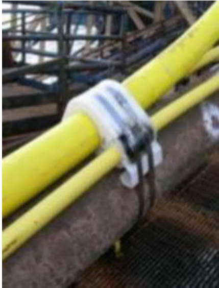
Figure 2: Piggyback clamp during construction/installation
