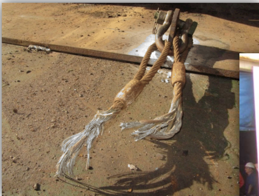
Failure of over-loaded wire rope sling
