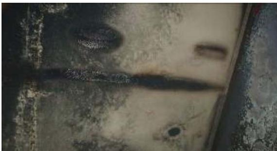
*Typical burnt paint from radiant heat associated with the welding on the main deck above*
