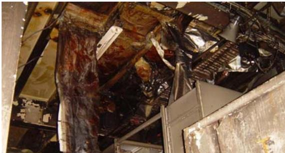
*Fire damage to the main store initiated from “flame washing” on the deck above.*
