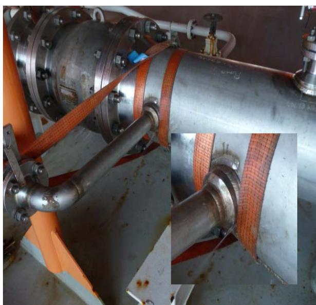
Seawater line with fatigue cracking
