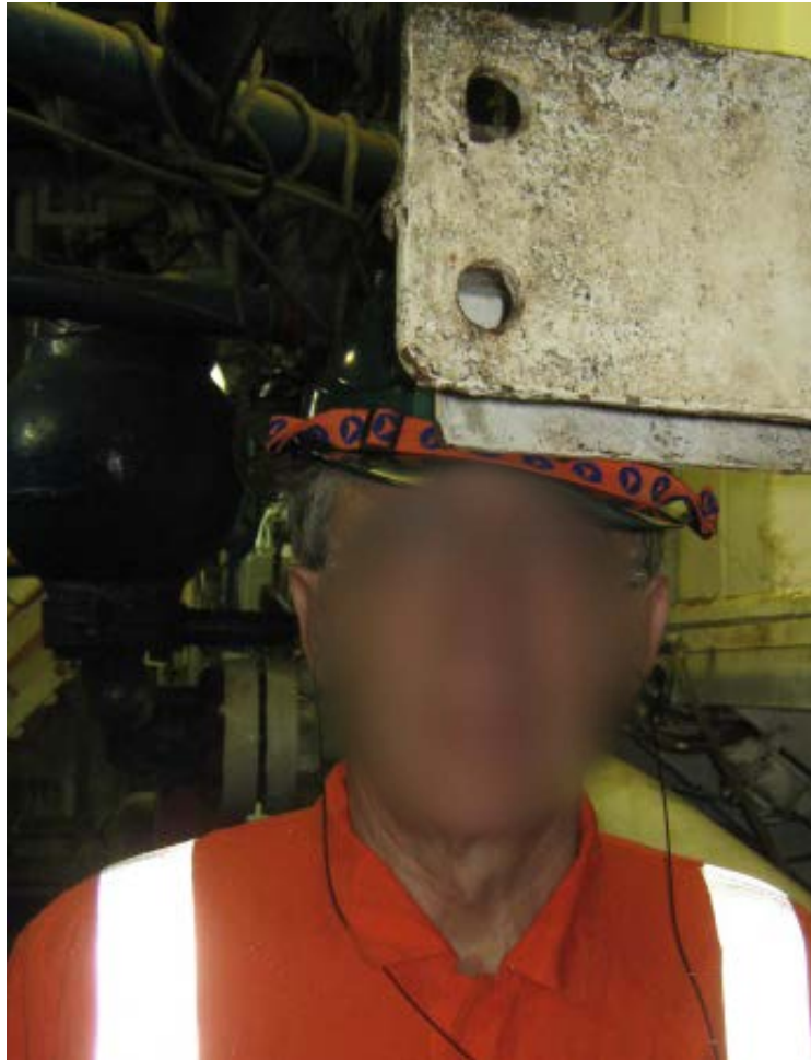
Figure 4 – Obstruction to escape route
