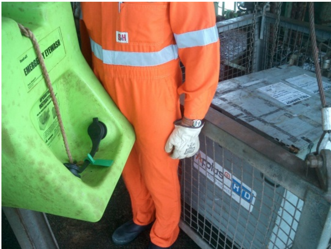
Figure 3 – Restricted access to eyewash station
