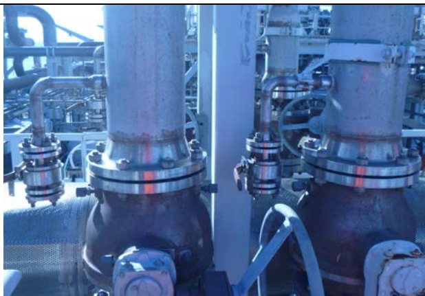
Figure 1 –Example of inconsistent bracing to deck SBC
